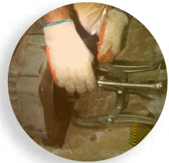
Escalator Motor Rehabilitation
