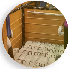
Elevator load test
