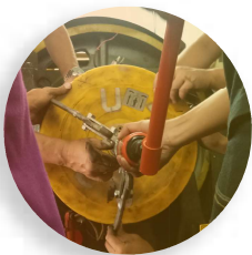
Elevator Motor Rehabilitation
