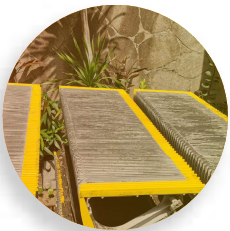
Escalator dirt and rust removal
