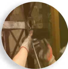
Elevator main rope replacement
