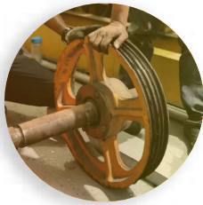
Elevator Bearing Replacement
