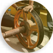
Elevator Bearing Replacement
