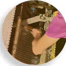
Escalator Step Chain Replacement
