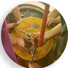
Elevator Motor Rehabilitation
