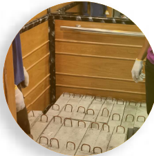
Elevator load test
