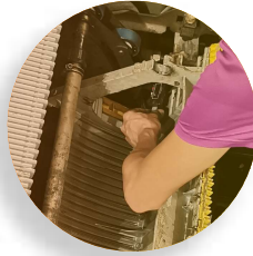
Escalator Step Chain Replacement
