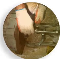
Escalator Motor Rehabilitation
