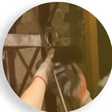
Elevator main rope replacement
