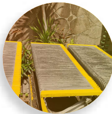
Escalator dirt and rust removal
