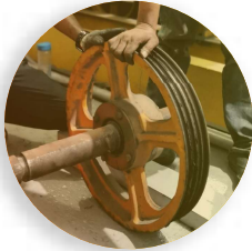
Elevator Bearing Replacement
